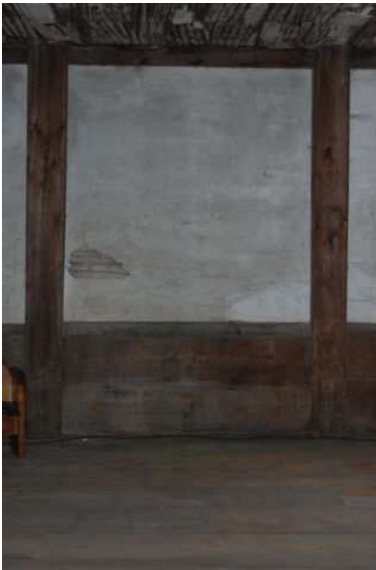
Interior view showing original (1769) posts and plate along eaves wall
