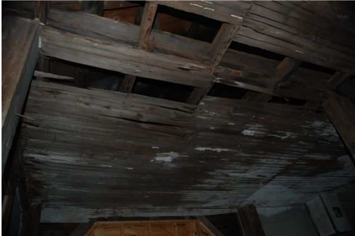
Detail of ceiling, showing split/accordion lath and joists
