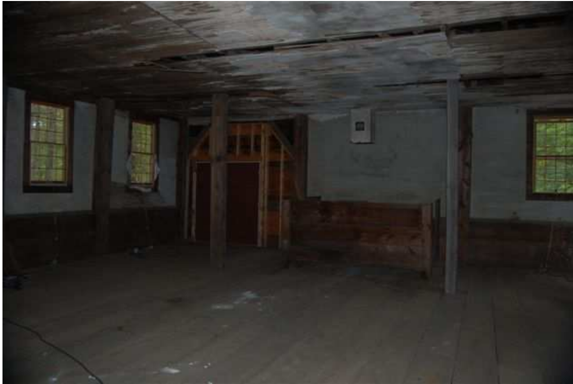
Interior view looking south showing southeast and southwest (rear) walls. Interior posts are not original. Wide opening in far corner was created for a barn-type door in 1912.
