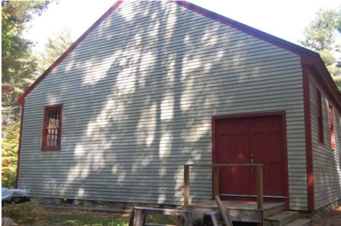
Detail of rear (southwest) elevation. Double doors date from late 1980s, installed to infill a barn-type opening created in 1912. After the building was cut down in 1838, there was a likely another window in the middle of this bay, placed similarly to that on the opposite gable end.
