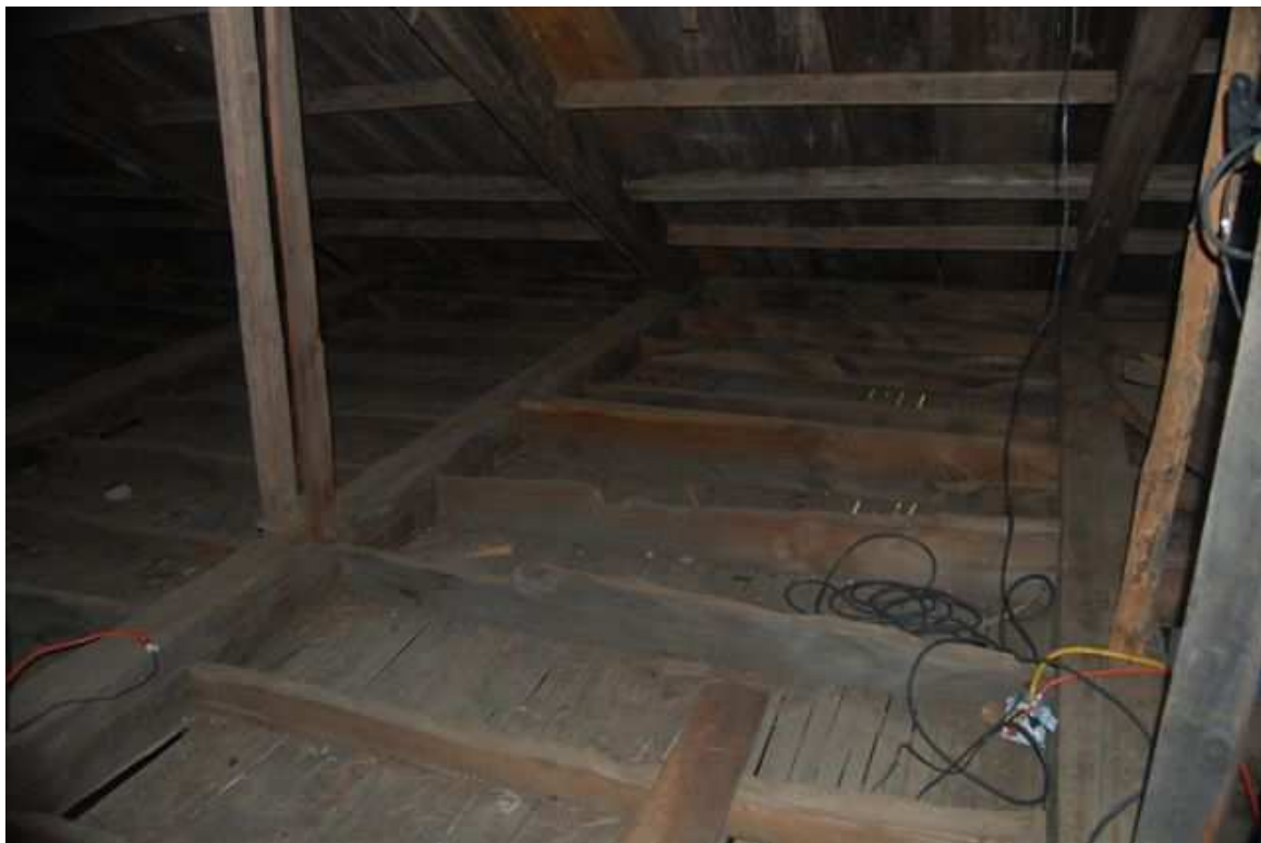
View of ceiling joists and lath, as seen from attic
