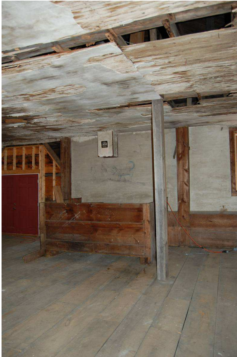
Looking southwest toward the moderator's box. Note also the ceiling joists, seen where the plaster has disengaged. Remains of the stove chimney can be seen in the center of this image, above the moderator's box.
