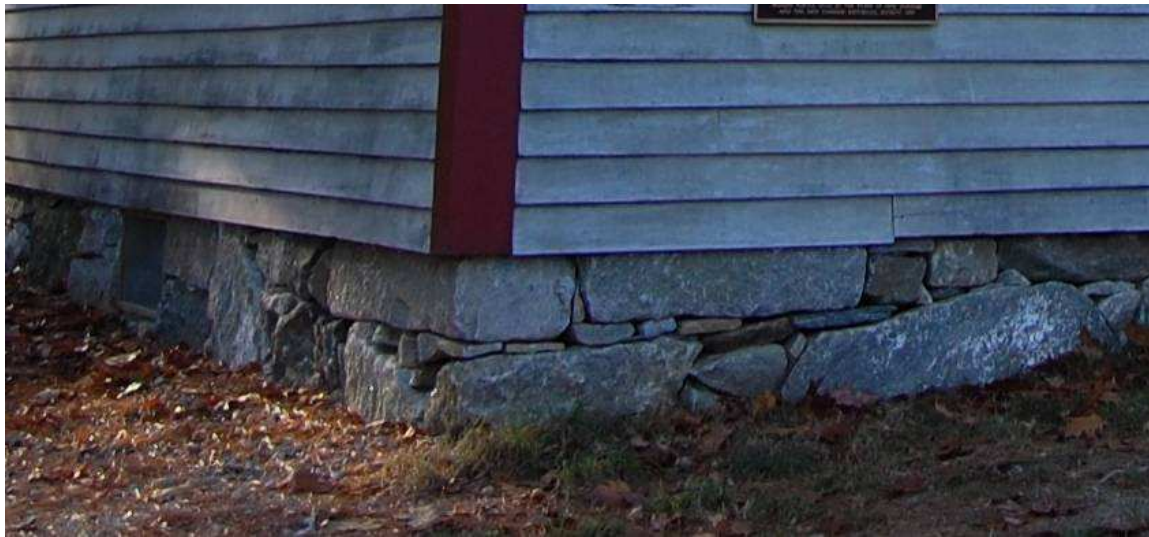
The east corner of the Meeting House showing the post-2006 foundation.
