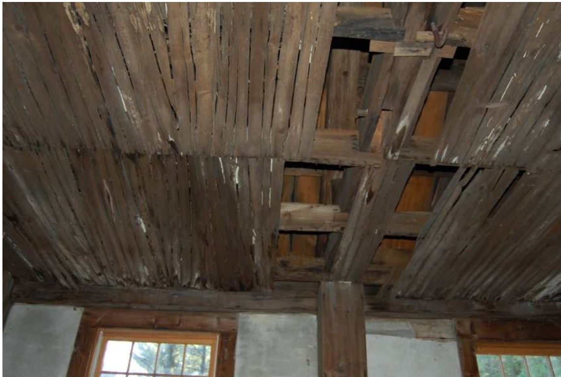
Looking up at the joists and lath of the ceiling, where the plaster has fallen away.
