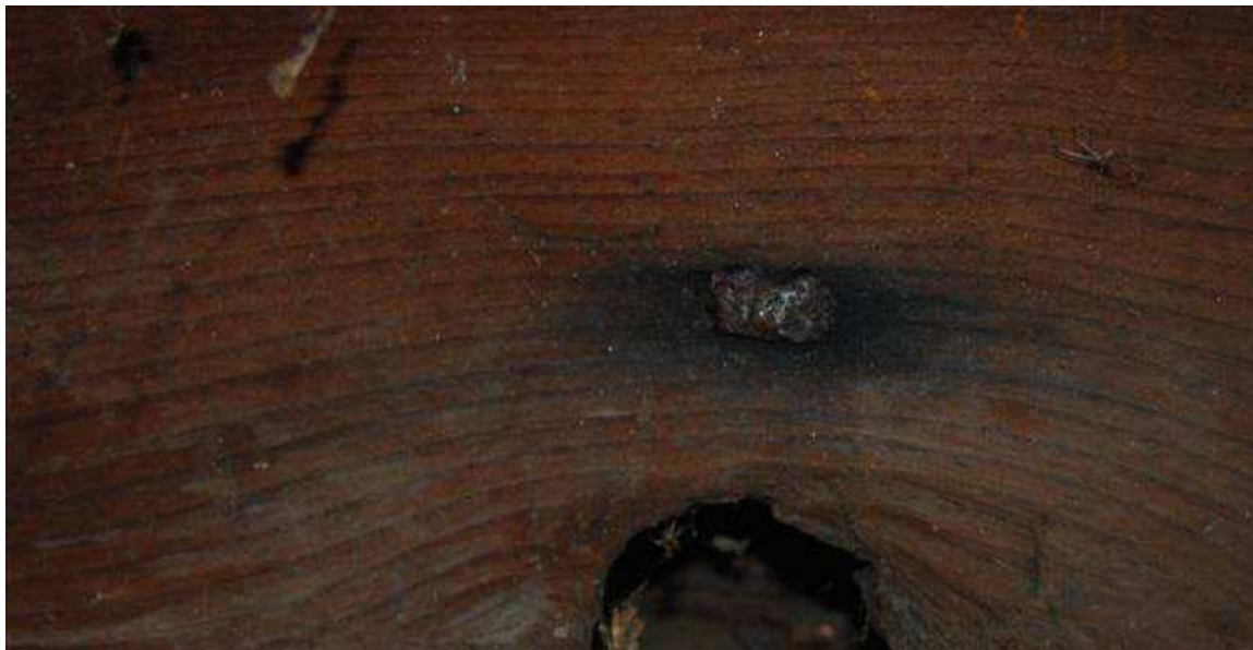
Detail of a butterfly, wrought iron nail in the wainscot
