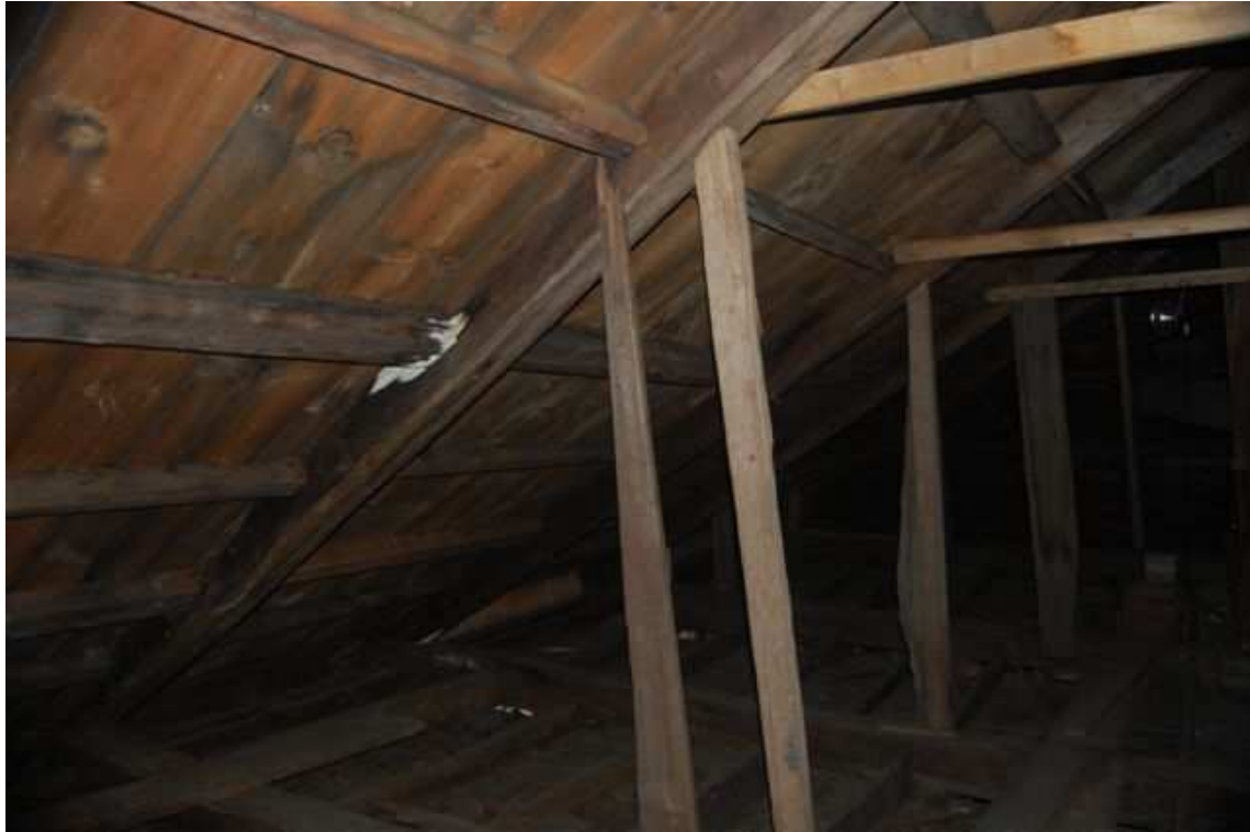
Attic roof system and bracing, with later additional bracing.
