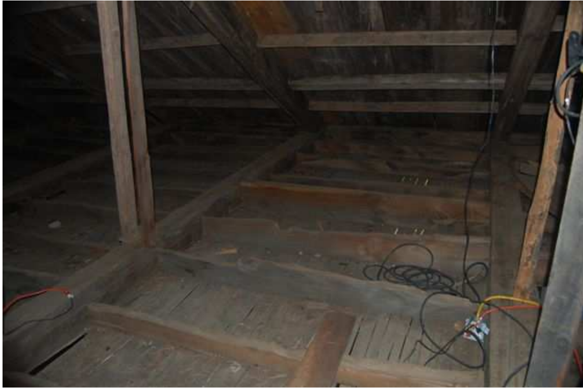
A view of the ceiling joists from above.
