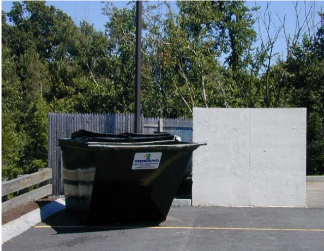
This trash enclosure was not properly sized to handle the dumpster needed for the facility.
