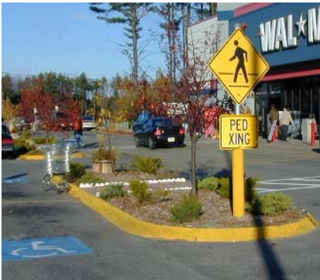
This internal walkway crosses over a curb, making access difficult for people with disabilities.
