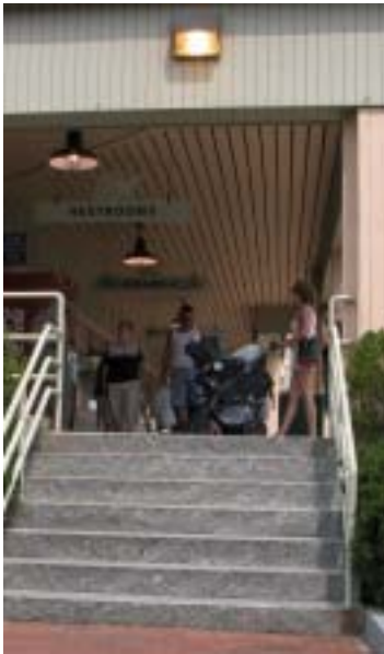
Unshielded wall-pac lighting can cause dangerous glare and make it difficult to see the stairway.
