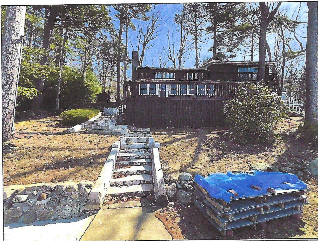
IMAGE 6 - 2 SUNSET LANE – NEW DURHAM, NH - APRIL 2, 2024 STANDING AT LAKE FACING EAST TOWARDS HOUSE
