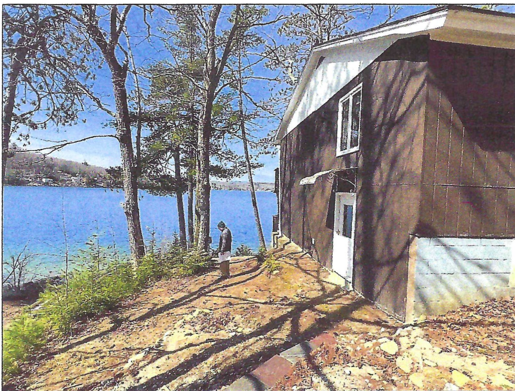
IMAGE 4 - 2 SUNSET LANE – NEW DURHAM, NH - APRIL 2, 2024 STANDING AT DRIVEWAY FACING WEST TOWARDS LAKE, SOUTH SIDE OF HOUSE
