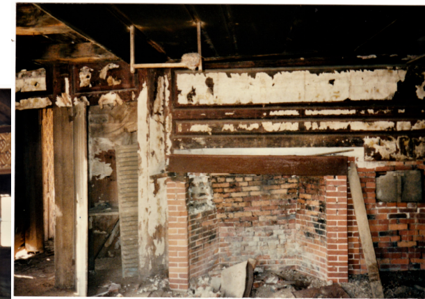
Photograph on the left is the parlor, on the right the East room fire place and bee-hive oven..
