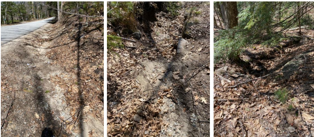
View of the stormwater ditch conveying runoff down the eastern road shoulder (left) to the culvert inlet (center) and to the culvert outlet on the west side of Kings Highway (right).
