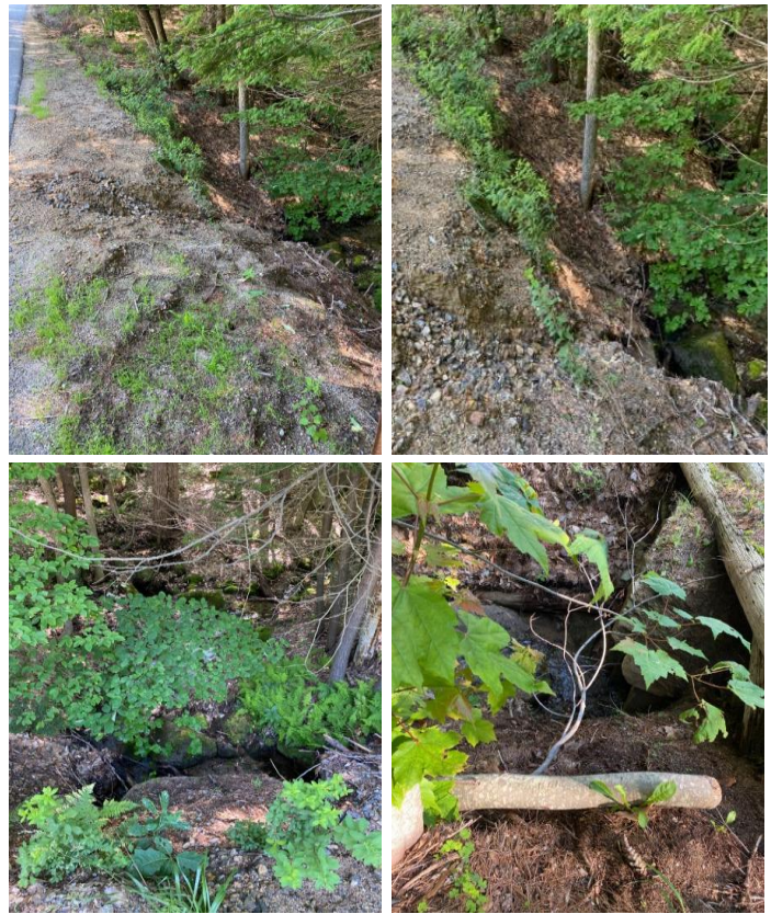
Top photos: Road shoulder erosion has caused a gully that flows directly into a stream. Bottom photos: The banks along the stream are unstable and easily eroded.
