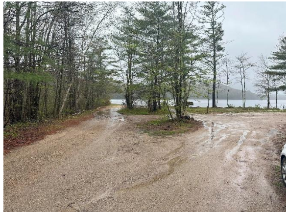
Photo 6: Lower portion of access drive, facing west. Note the eroding flow paths along the drive. The driveway to 234 Kings Hwy is to the right (north).
