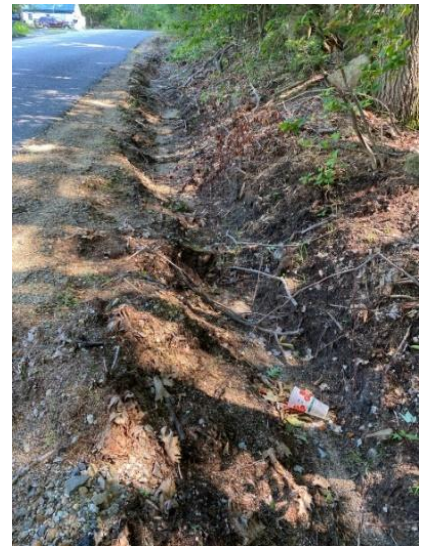
Road surface and shoulder erosion on Kings Hwy (Site 1-10).
