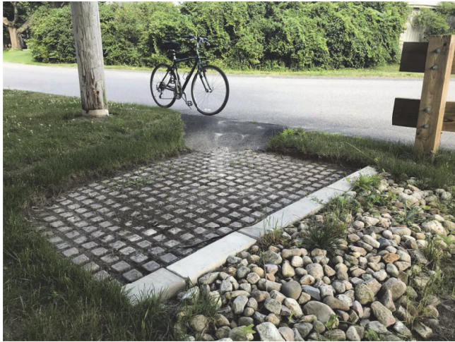
Sediment forebay with paver mat
